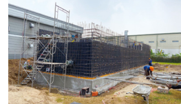
Construction of a fire extinguishing tank for the sprinkler system
