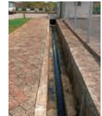
Completely cleaned gutters
