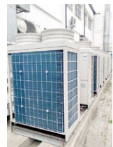
New air conditioner external unit
