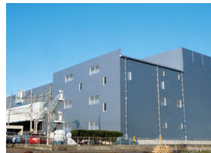
New building for producing optically function films (Shingu Plant)
