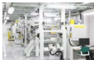
Large-scale pilot coaters in the Advanced Technology Building
