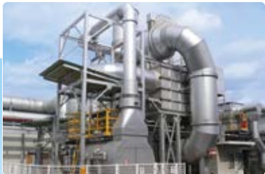
Waste heat boiler
