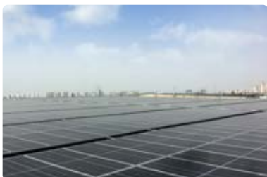
Solar power generation system
